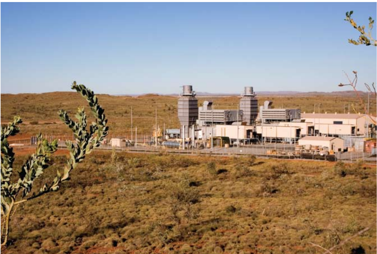
The new Karratha Power Station.
