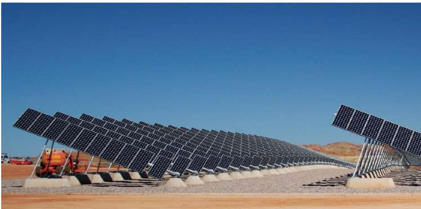
Marble Bar Pippunyah solar-diesel power station.
