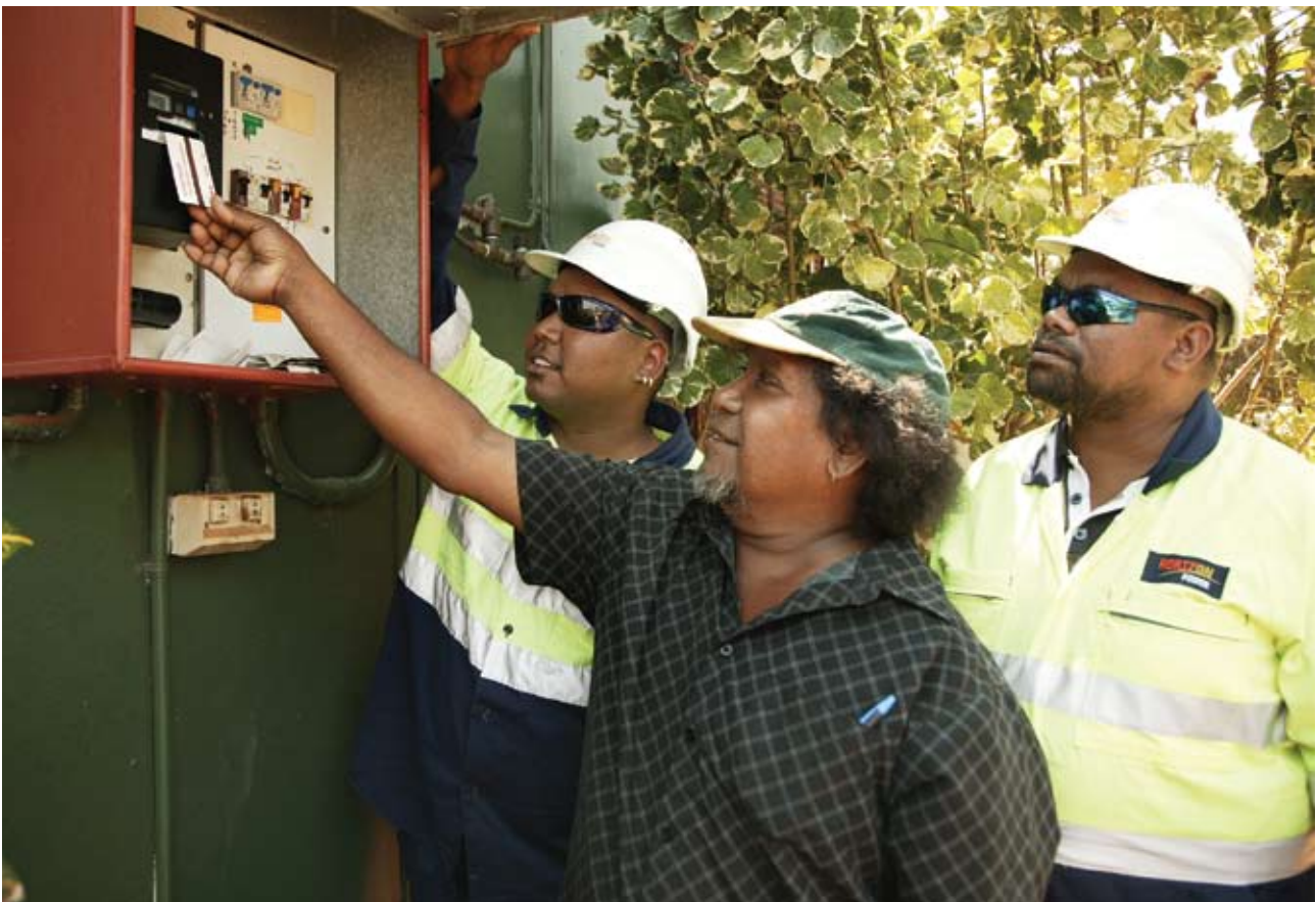
Prepayment meters have brought significant advantages to remote communities.
