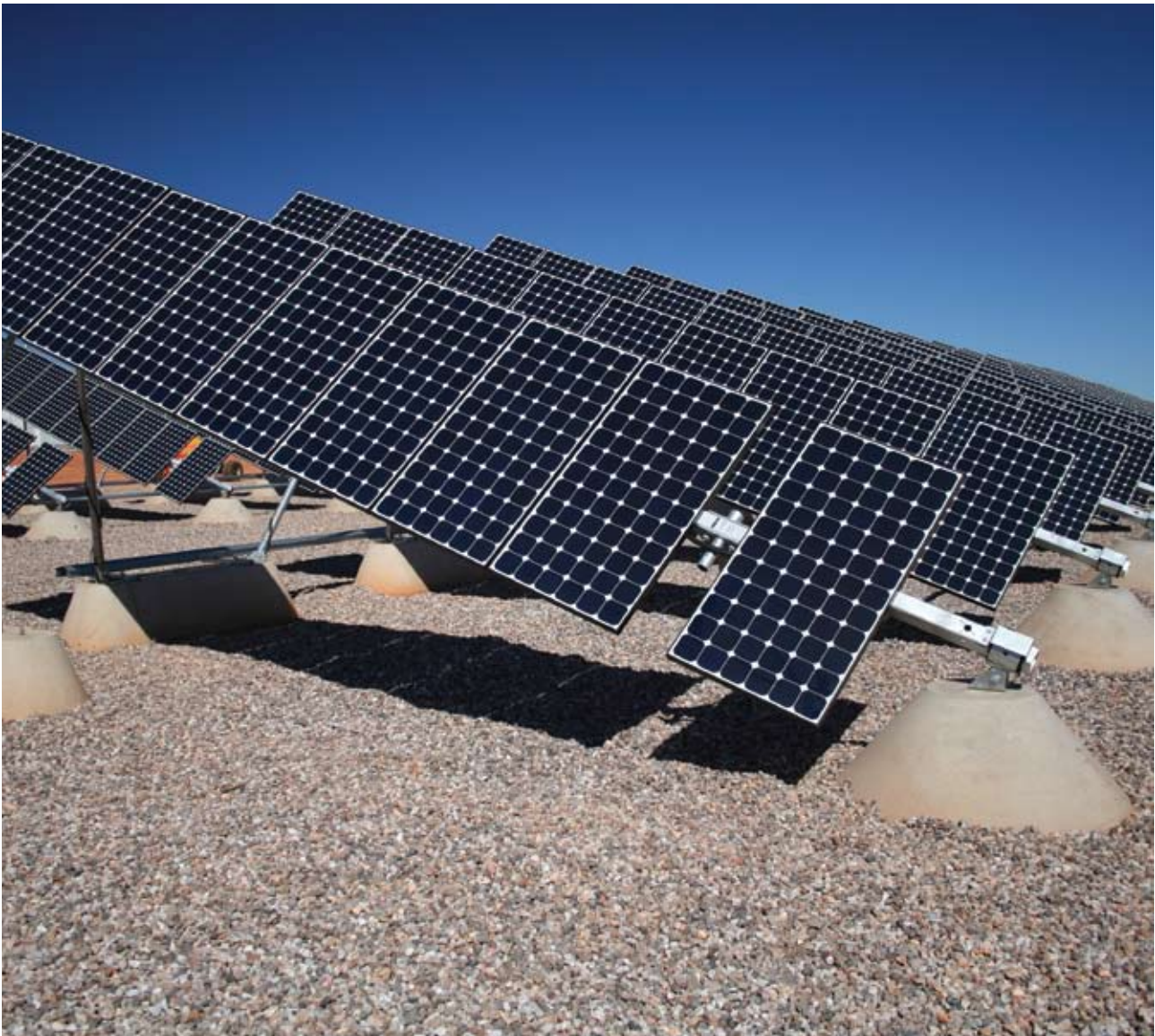
Solar panels, Marble Bar Pippunyah solar-diesel power station.
